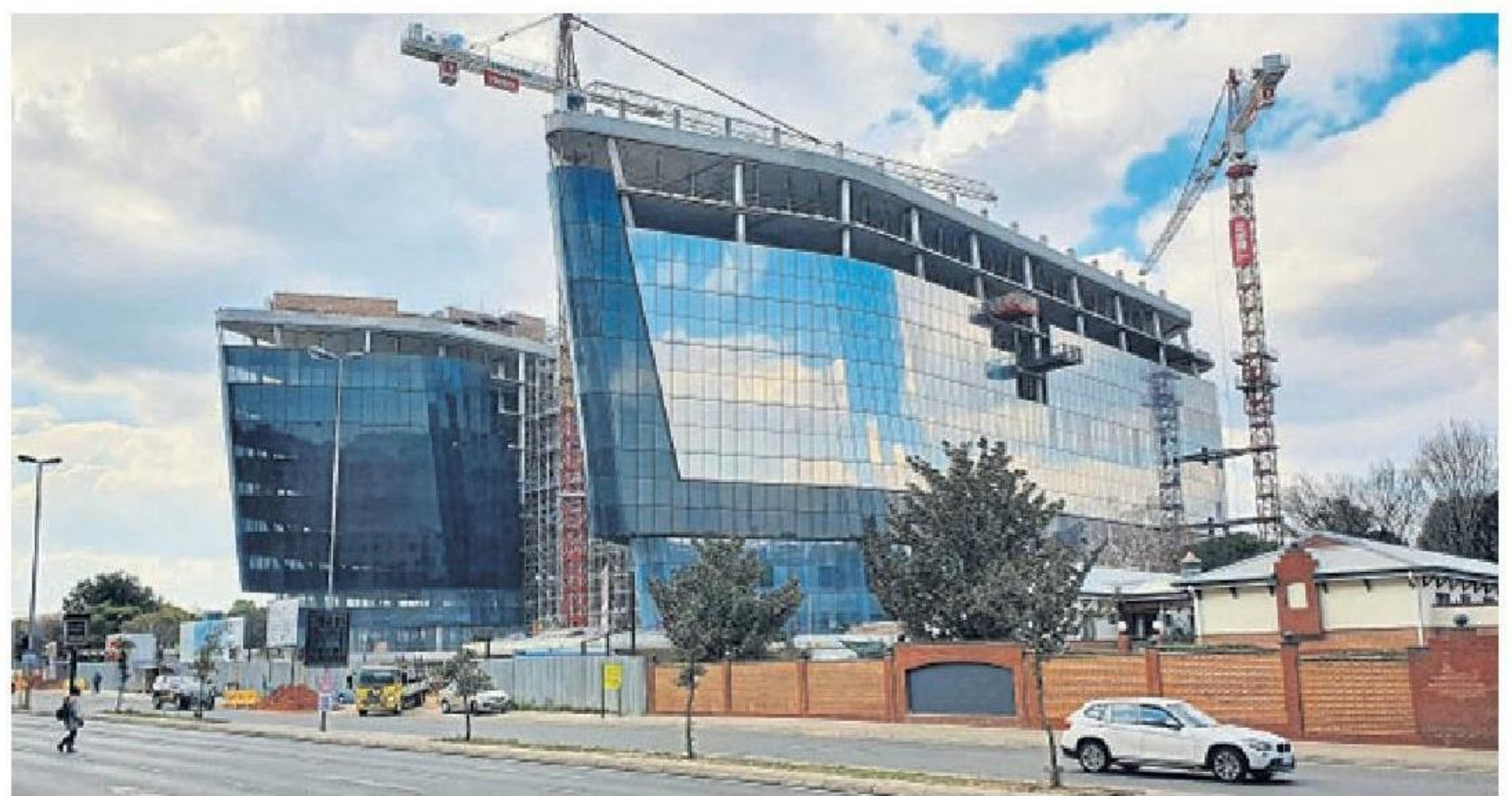
Premium: Growthpoint's new office development in Rosebank, 144 Oxford. /Alistair Anderson
