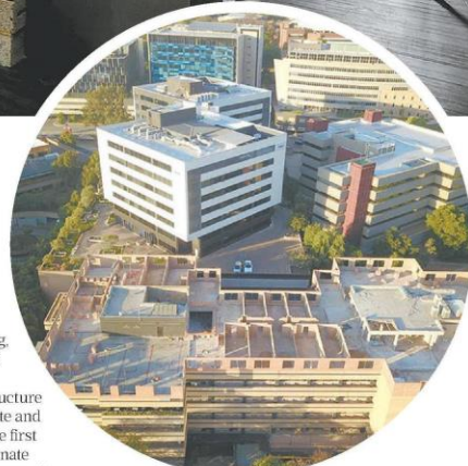
Black Brick before the refurb
