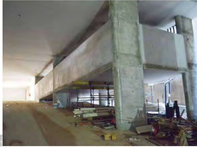
There are two basement parking levels and five parkade levels.
