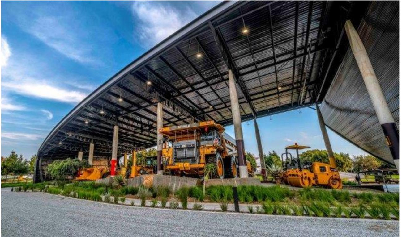
While the shape provided the volume and extent that such a showroom required, it also posed a range of structural challenges. The integrity of the ‘bubble’ design was ensured by maximising the grid distance and using steel as the main structural element.
