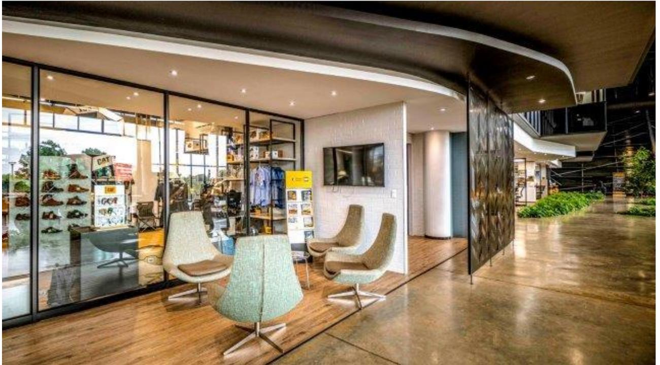
The flush-glazed unitised façade with performance-glass affords the main view into the showroom. An important benefit of the ‘bubble’ shape is that the canopy of the top edge has a 3.5 m cantilever, which not only gives excellent shading in summer, but is exposed in winter, which heats the internal space naturally.
