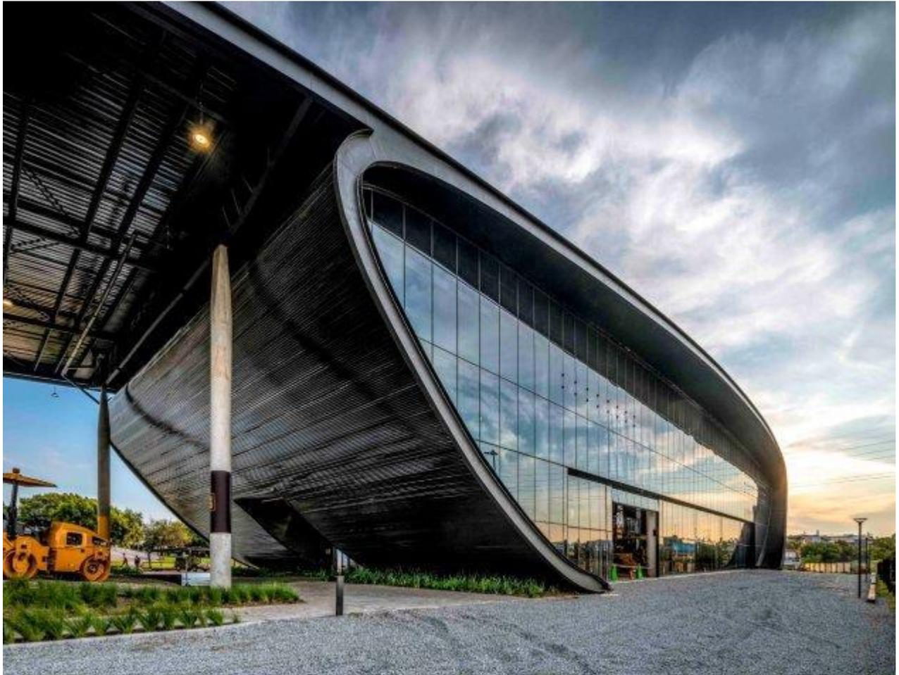
A steel girder framework provided the tracked-shape design of each of the two bubbles, with large spanning trusses carrying the roof, all sitting on a specially-devised grid to accommodate the different sized equipment required. The two ends of the building consist of curved structural steel and horizontal sheeting that both cantilever 15 m out from the base and are 15 m high.
