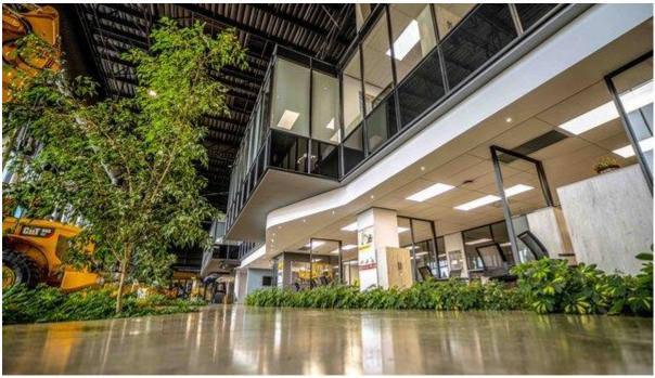
The award-winning Barloworld and Caterpillar Head Office and Showroom in Isando This presented an engineering challenge to keep the deflections within allowable limits while also keeping the structural elements economical and within the allowed sizing envelope, especially since the large cantilevered bowing also carried a flushed glazed façade with stringent allowable deflections. Stressed cables were used to hang the bowing cantilevered arches from the remainder of the roof.
