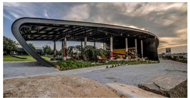
The 3 200 m2 showroom 'bubble' was built to face directly onto the R24 A steel girder framework provided the tracked-shape design of each of the two bubbles, with large spanning trusses carrying the roof, all sitting on a specially-devised grid to accommodate the different sized equipment required. The two ends of the building consist of curved structural steel and horizontal sheeting that both cantilever 15 m out from the base and are 15 m high.
