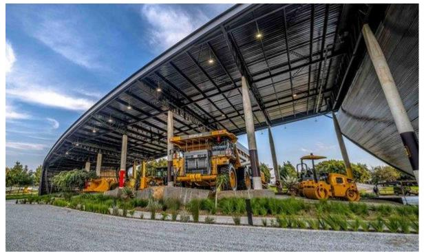
The integrity of the bubble design was ensured by maximising the grid distance and using steel as the main structural element
