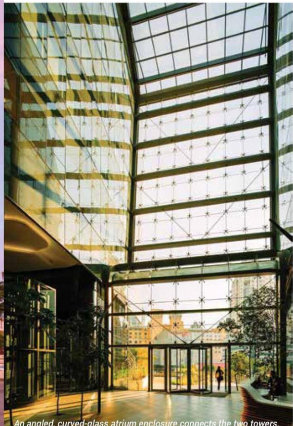
An angled, curved-glass atrium enclosure connects the two towers.
