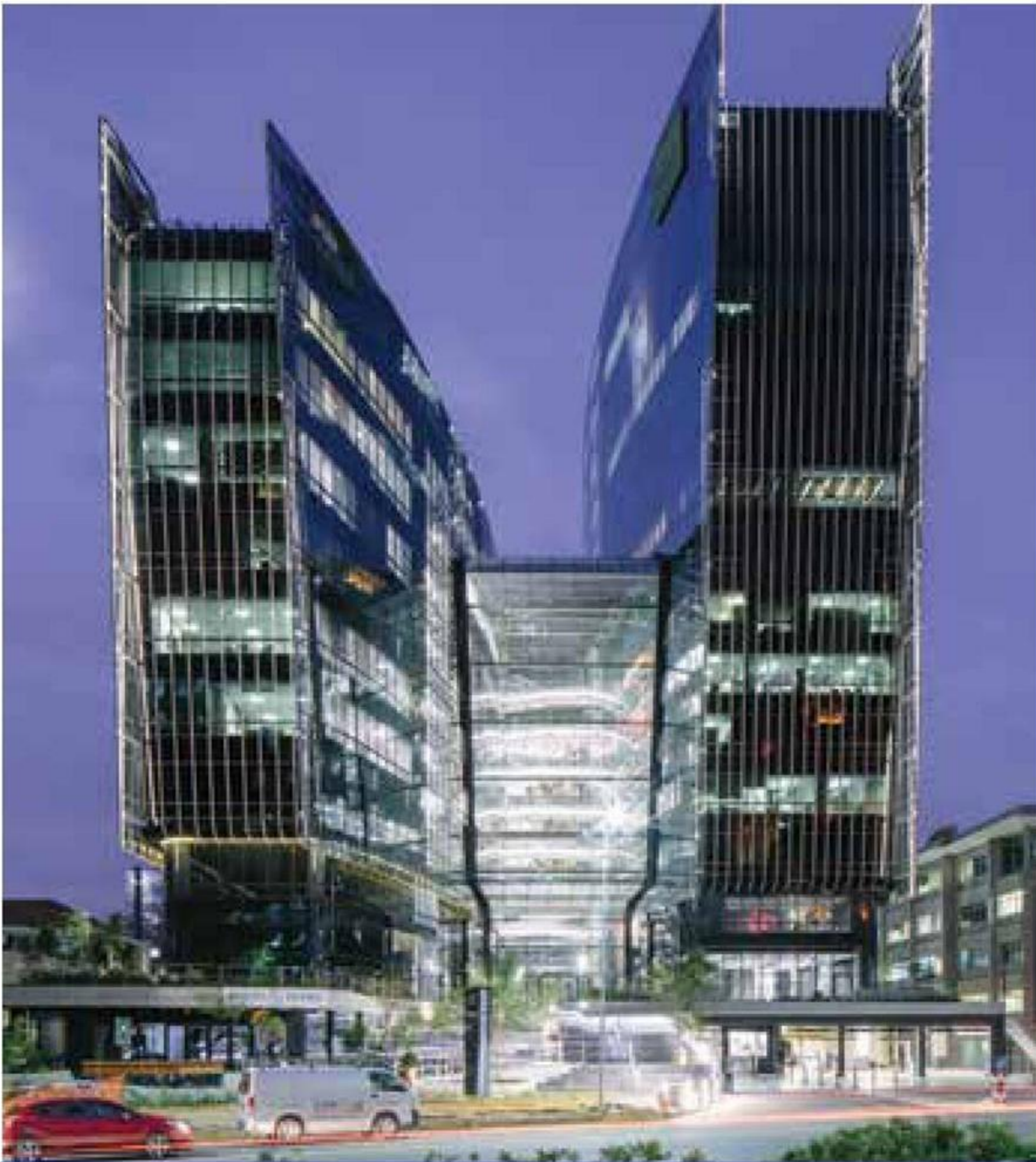
The main architectural feature is the curved glass atrium connecting the two towers
