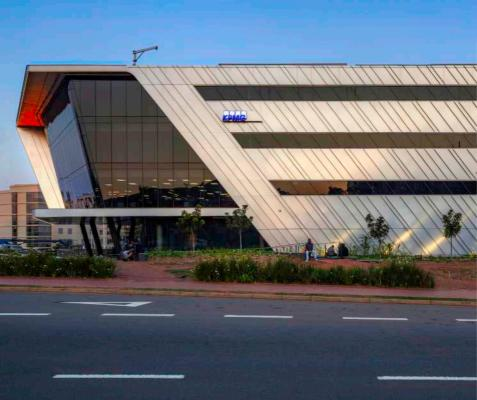
Known as Pran Boulevard, the development consists of two separate office buildings of three levels, each above ground floor, linked together on each level with enclosed glazed bridges. There are three parking levels providing about 250 parking bays, as well as a ground-floor podium level with timber decks, walkways, landscaping, and water features. The total building area, including the parking levels, is about 18 600m<sup>2</sup>.
