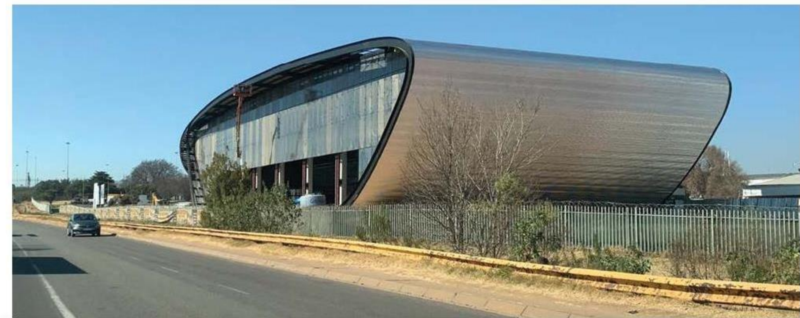
The Barloworld CAT Equipment Showroom takes shape
