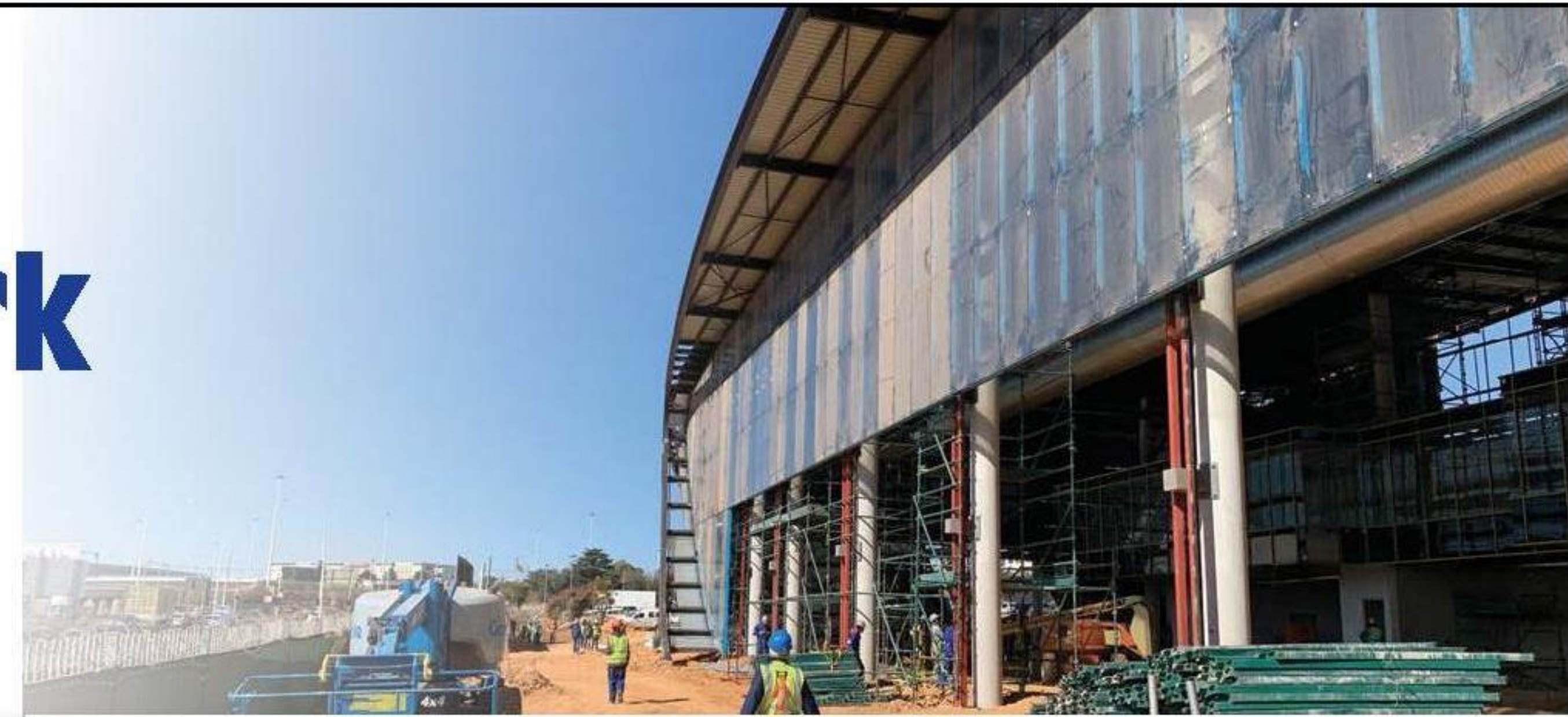
The steel structure was extremely difficult to manufacture and to erect
